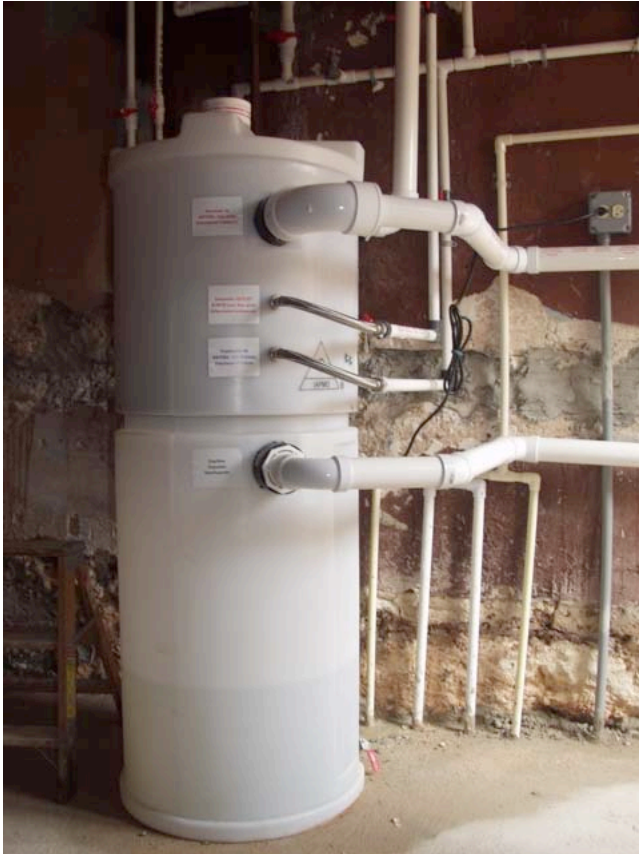
Grey water system installed
